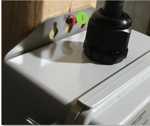
Figure 41 : Sheet metal screws on wooden stake for installation of a vacuum transmitter
