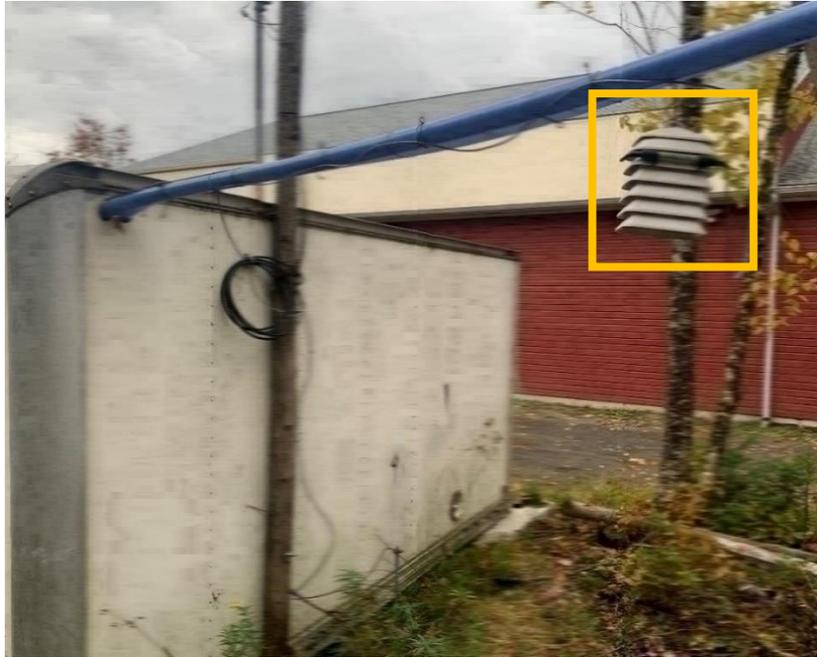
Figure 92 : External temperature sensor installed
