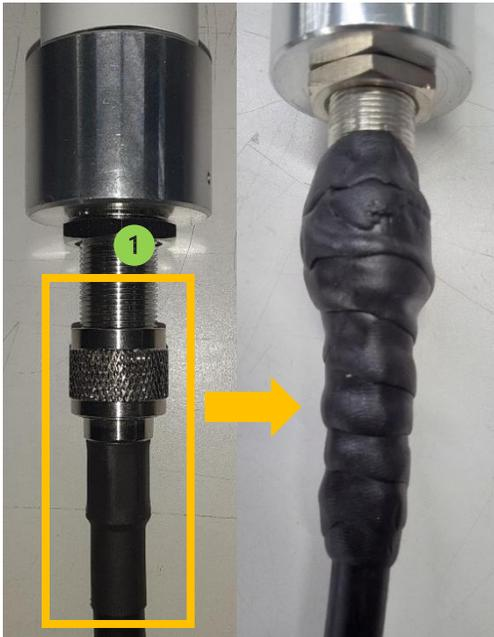
Figure 100 : Antenna Coax-seal option B or C
