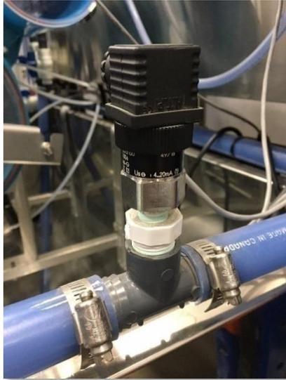
Figure 58 : Screw-in pressure sensor installed
