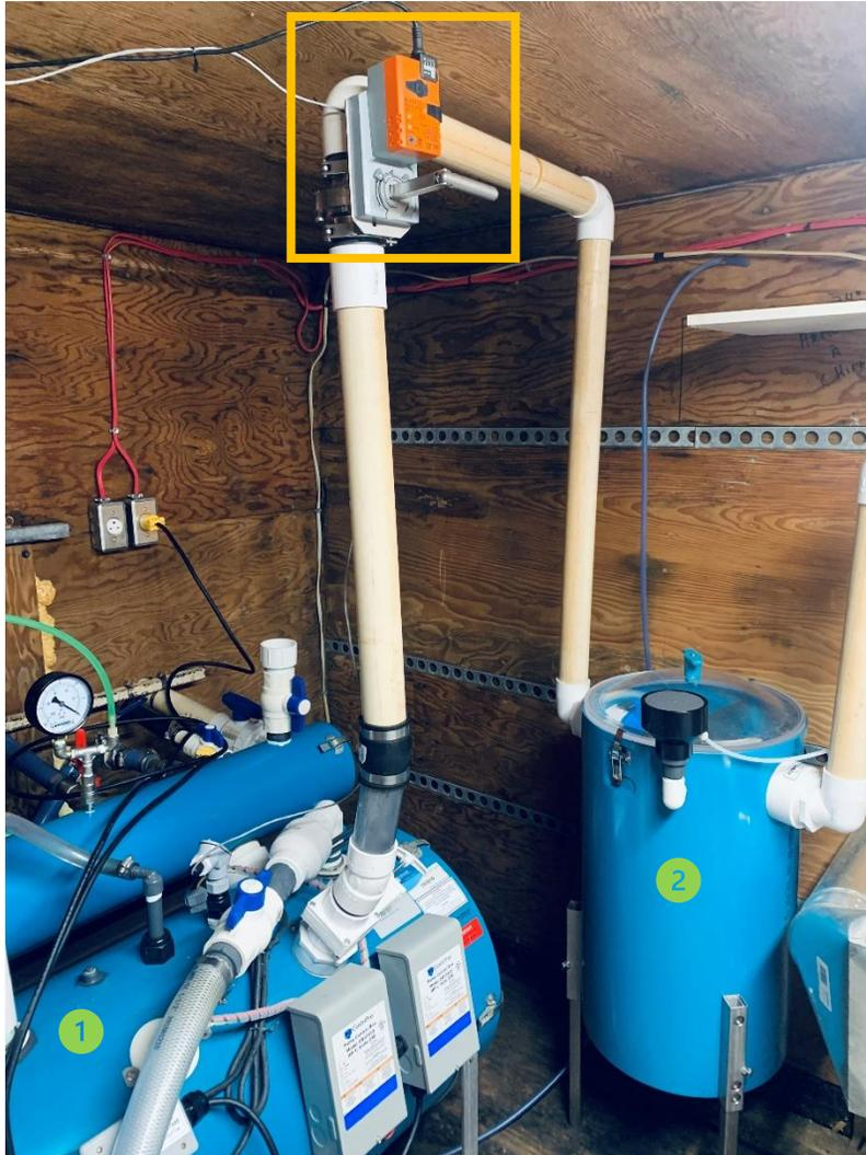
Figure 77 : Vacuum modulation valve installed
