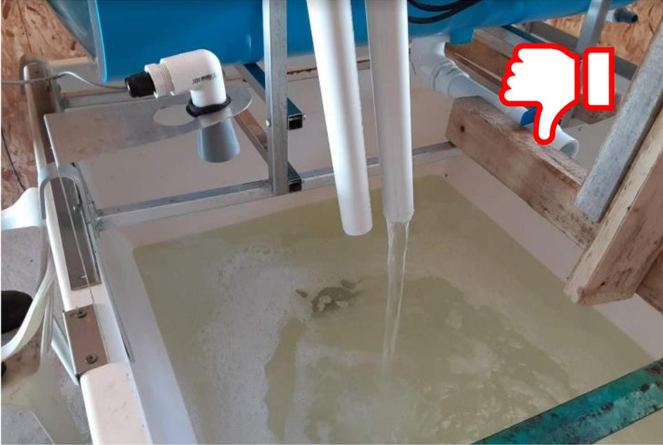
Figure 53: Ultrasonic tank level sensor not properly installed
