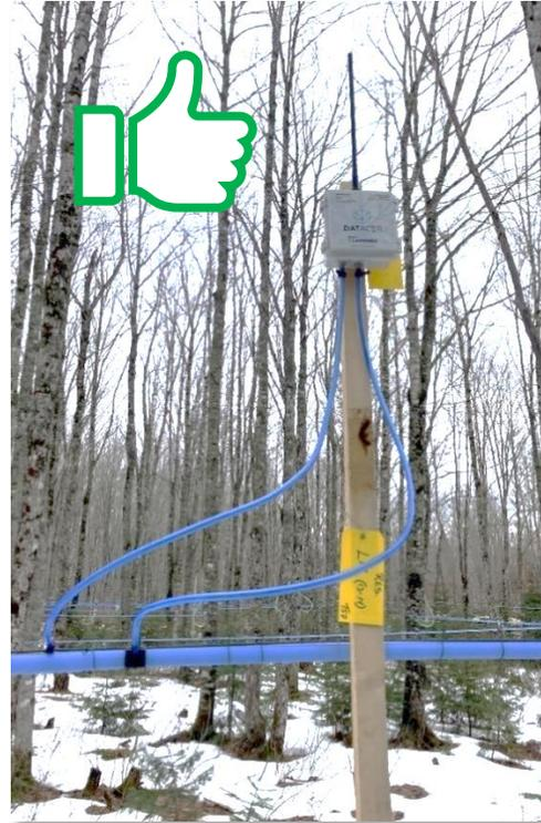
Figure 43 : Vacuum transmitter properly installed
