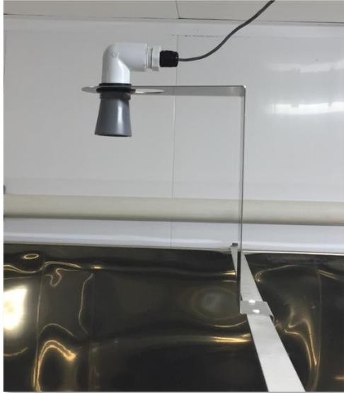
*Figure 51 : Tank level sonar sensor installed*
