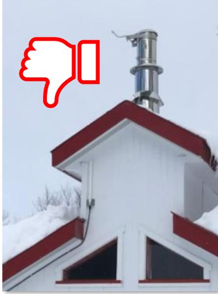
Figure 98 : Antenna on a building improperly installed
