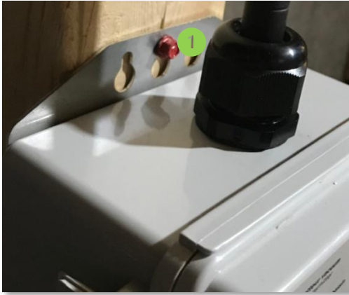
Figure 46 : Sheet metal screws on wooden stake for installation of a vacuum transmitter
