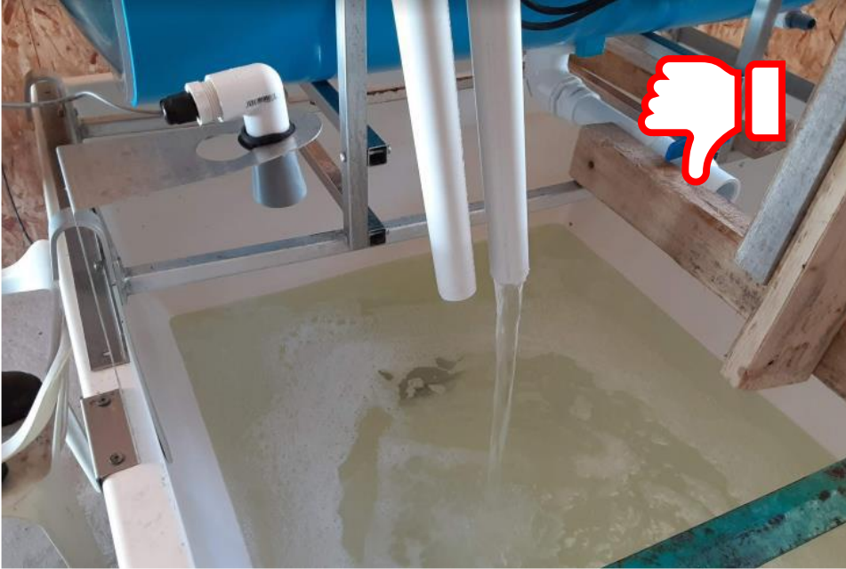
Figure 59: Ultrasonic tank level sensor not properly installed
