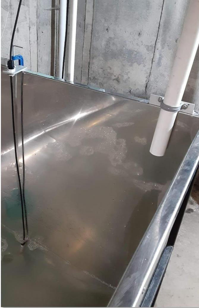
Figure 65: Submersible sensor installed
