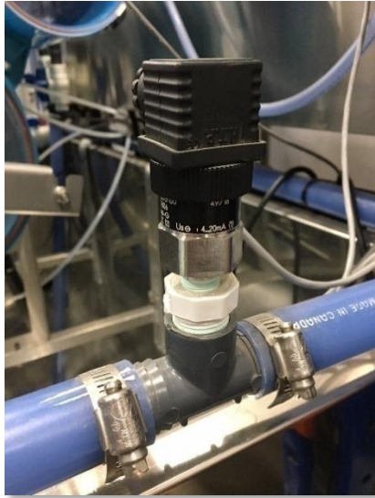
Figure 64 : Screw-in pressure sensor installed
