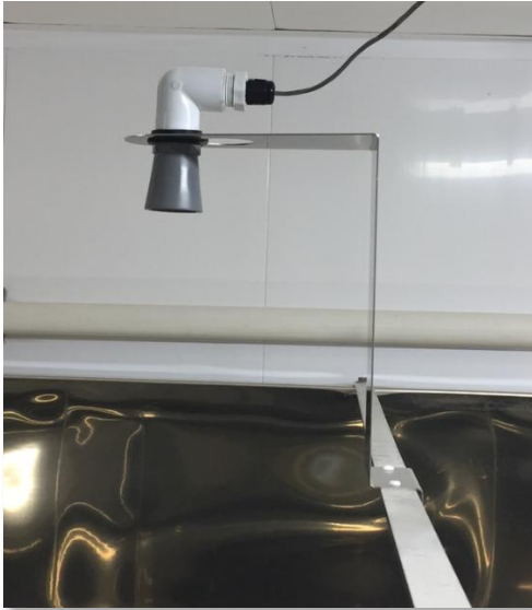
Figure 57 : Tank level sonar sensor installed
