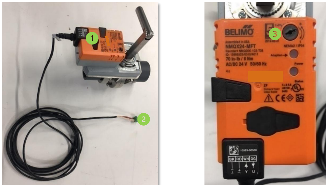
Figure 11 : Vacuum modulation valve
