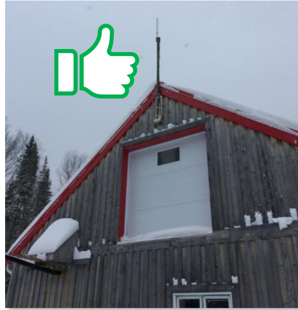
Figure 121 : Antenna on a building properly installed
