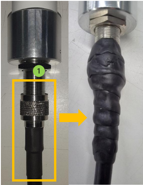
Figure 122 : Antenna Coax-seal option B or C
